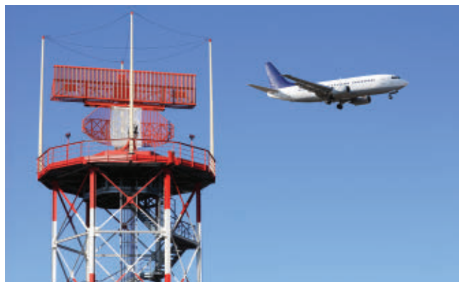
▲ Fig. 2 Airport co-located primary and secondary radar system. The SSR radar antenna is at the top with the S-Band antenna immediately beneath it. (Photo courtesy of Shutterstock.com).
